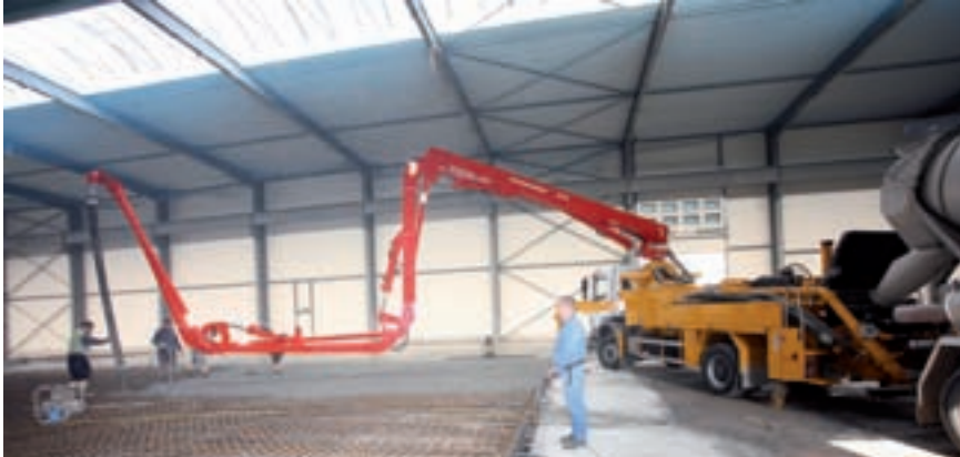
Superior performance when concreting in low buildings – thanks to low unfolding height and flexible roll-Z-fold system
