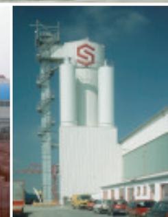
Liebherr-mixer system combined with a block manufacturing plant.
